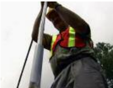
Threading the ShapeAccelArray into the ground
