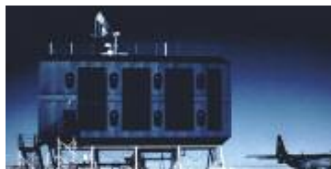
SolarWall™ John Hollick, 1995 installed in over 25 countries, from Wal-Mart stores to a research station in Antarctica.
